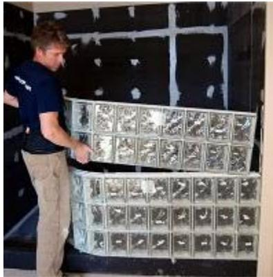
**4.** Place the second panel on top of the first and push into the wall until the vertical joints line up. (Tip...if the second panel is hitting the anchor at the wall and the vertical joints don't line up; pry the first panel out away from the wall until they do.) Repeat steps on all sections but the top panel.
