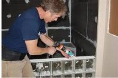
**3.** Apply two-1/4" beads of silicone to the top of the spacer on the first panel and a 1/2" bead to the wall to the height of the second panel.
