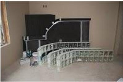
**1.** Your modular glass block wall will arrive as separate components. In addition to the glass block wall, you should also receive a 'Split Kit' that contains silicone for gluing the panels together, Panel Anchors for attaching the modular sections to the wall at the jamb, and grout for finishing the face joints. The kit shown here also incorporates a wedi® Ready 4 Tile® shower pan and wall system.
