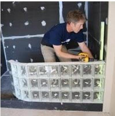
**2.** Install panel anchors into top horizontal spacer on each modular wall section, except for the top panel. Run 1/2" bead of silicone at centerline of where panel will sit on the curb, and a 1/2" bead of silicone up the jamb to the top of the base panel.
